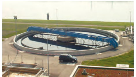
▪ HIK Doppel-Rundschildräumer / HIK double circular-tank shield scraper
